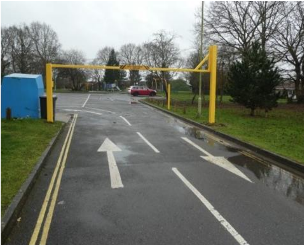
New Car Park Barrier erected by Fareham Borough Council.
